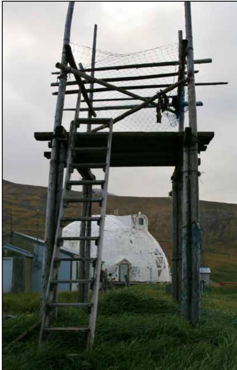
Figure 12. A Wales storage platform and drying rack constructed of driftwood.
